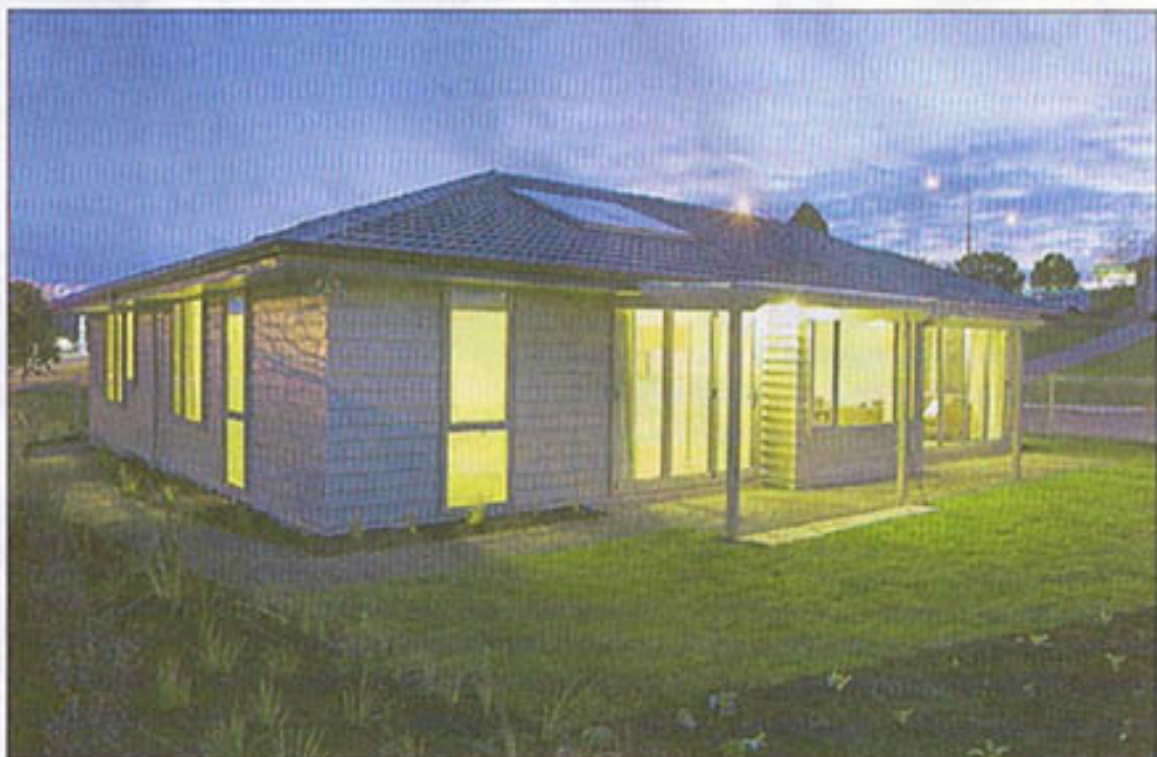
The Now Home, Waitakere City, Auckland: looks conventional, but incorporates many energy-saving features at no extra cost. Photo: Craig Robertson
