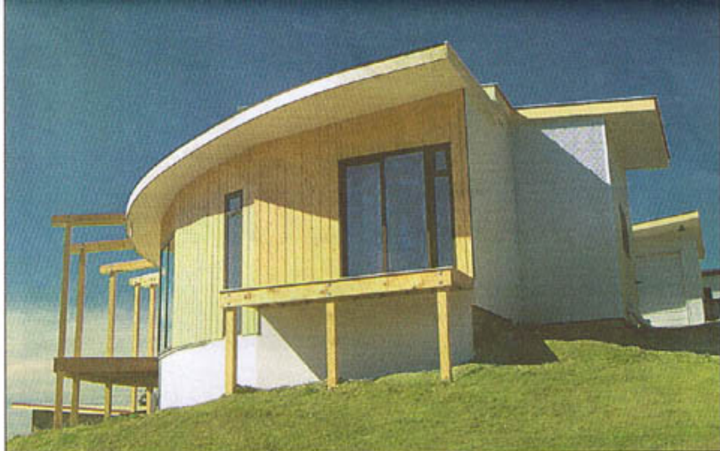
Versatile comfort: architect Helen Richard's Nelson home uses thermal mass in the form of solid concrete walls and floor to store energy. Despite the weather, it maintains an even temperature, slashing energy bills.
